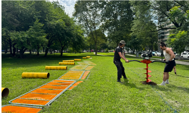
Bar None installation in Maja Park at 22nd street on the Parkway.
